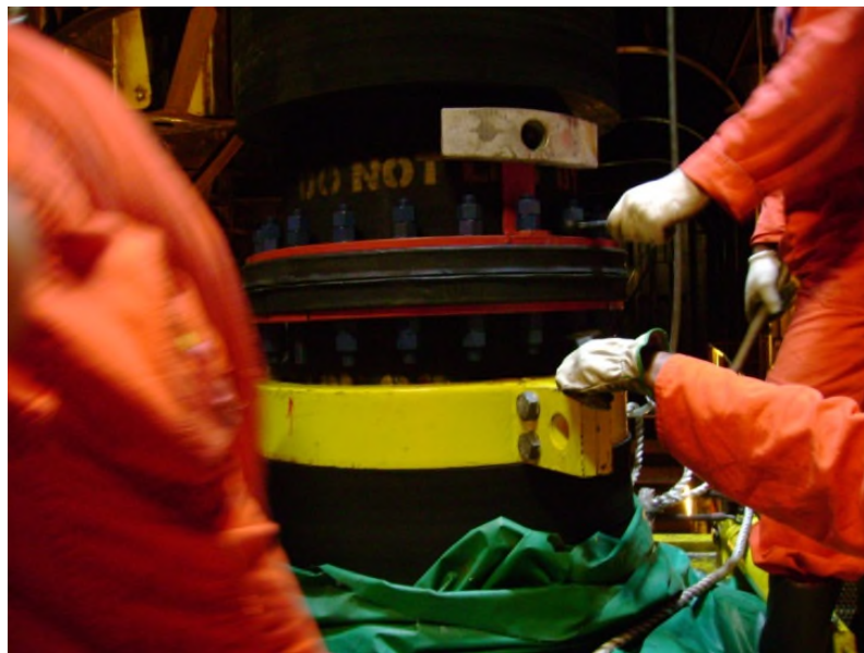
Fig.2-15: Flange Connection with Carbon Steel Stud bolts & Anodes
