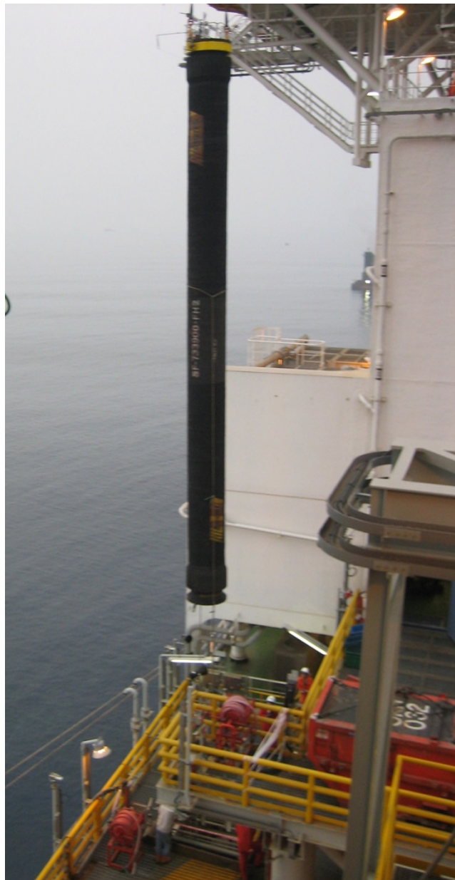
Fig. 6: Flexible Pipe Section
