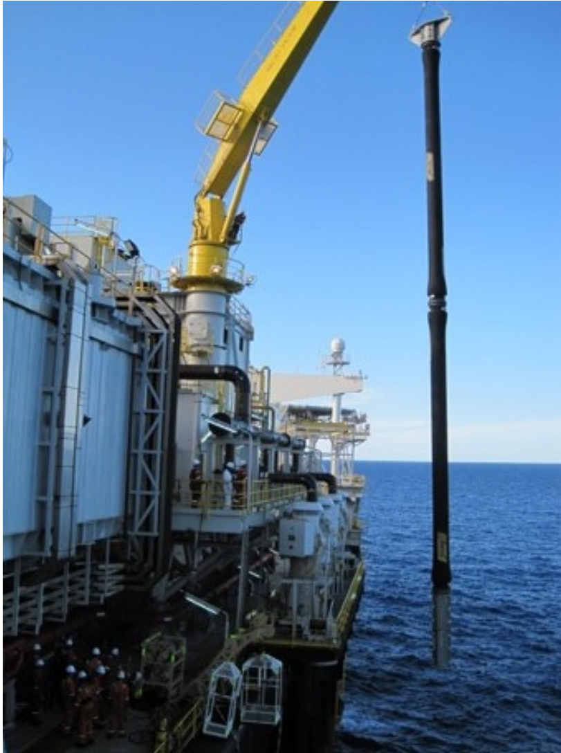
Fig. 11: Assembled Flexible Pipe String being lowered overboard for a Diver Assisted Installation
