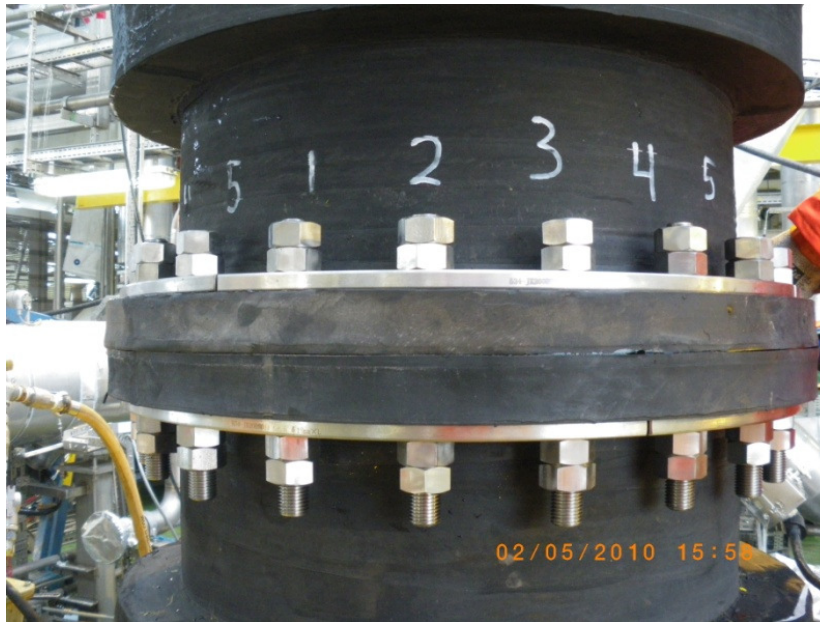
Flexible Hose Connections: Titanium Bolting / Backing Quadrants Hose flanges encapsulated with Rubber No exposed CS in Hose Section
