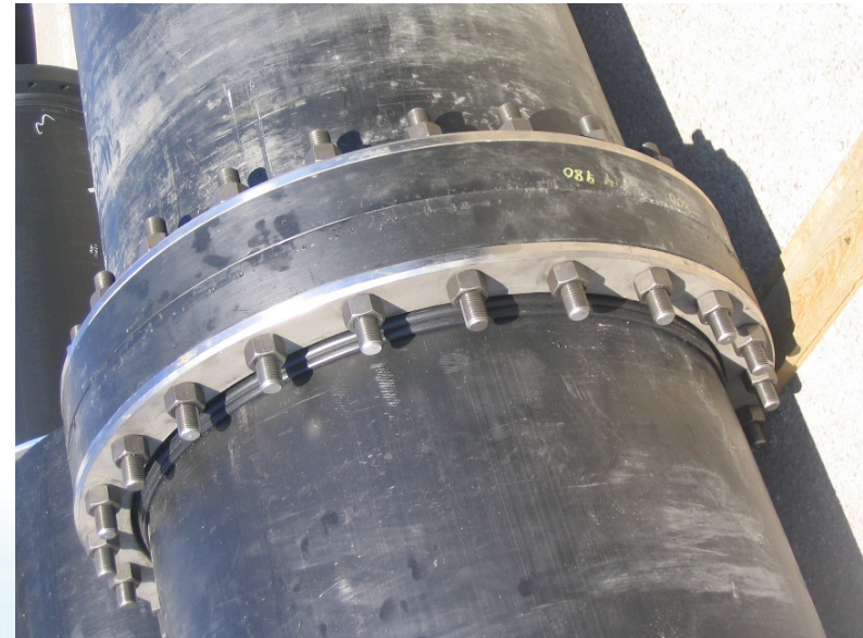
HDPE Connection: Super Duplex Bolting / Backing Rings HDPE Corrosion Resistant
