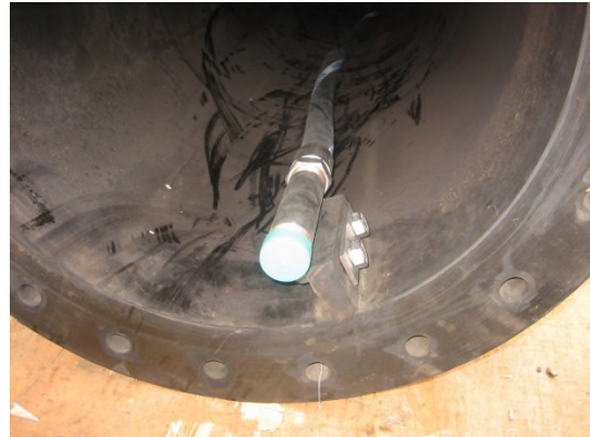
Fig. 7: Hypochlorite Line
