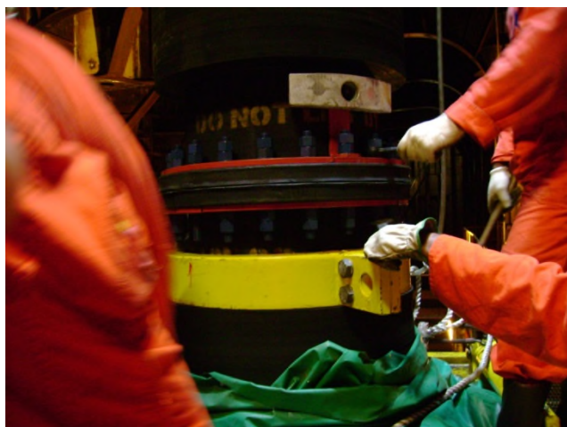
Fig. 16: Flange Connection with Carbon Steel Studbolts & Nuts and Anodes
